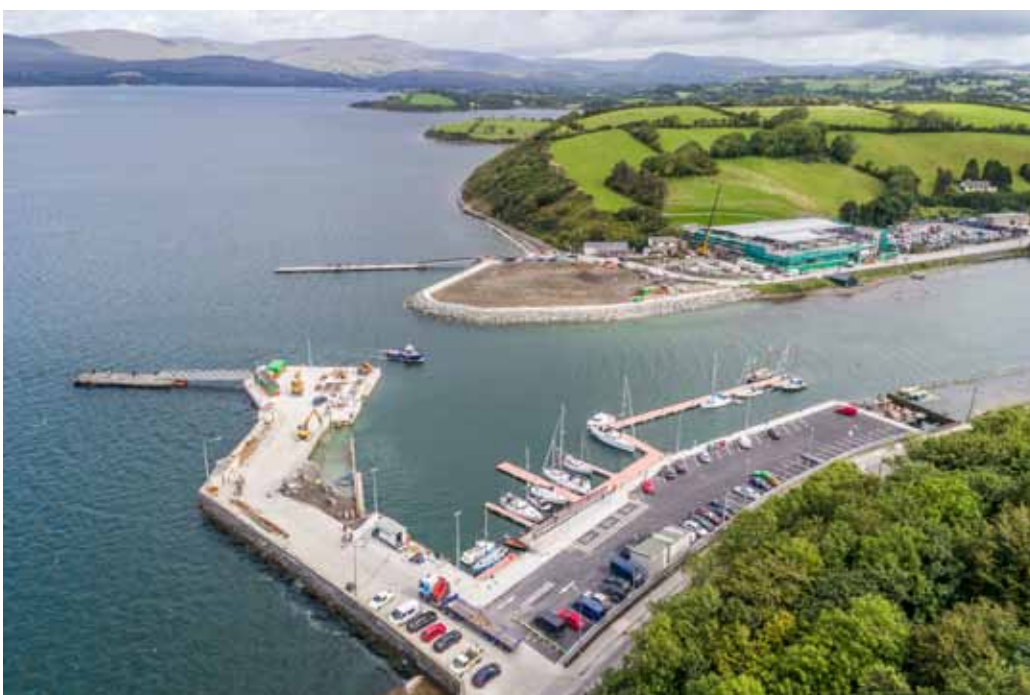
View NE over Bantry Harbour showing the new marina, the extensions to the Town Pier and the reclaimed land opposite (Bantry Bay Port Company)
