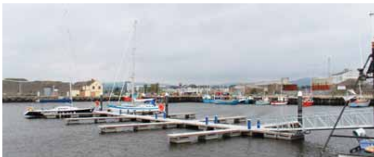
The new pontoons in the dock at Arklow
