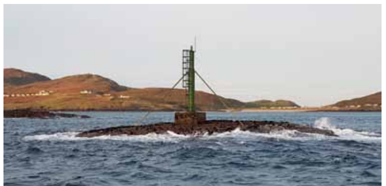
Bar Rocks new beacon, from the E (Donegal County Council)
