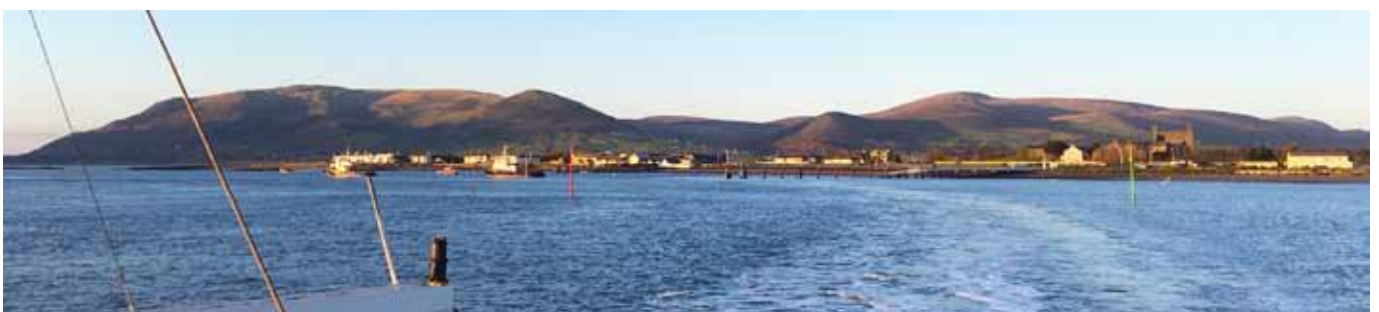
Greencastle ferry terminal and new perches, from the S
