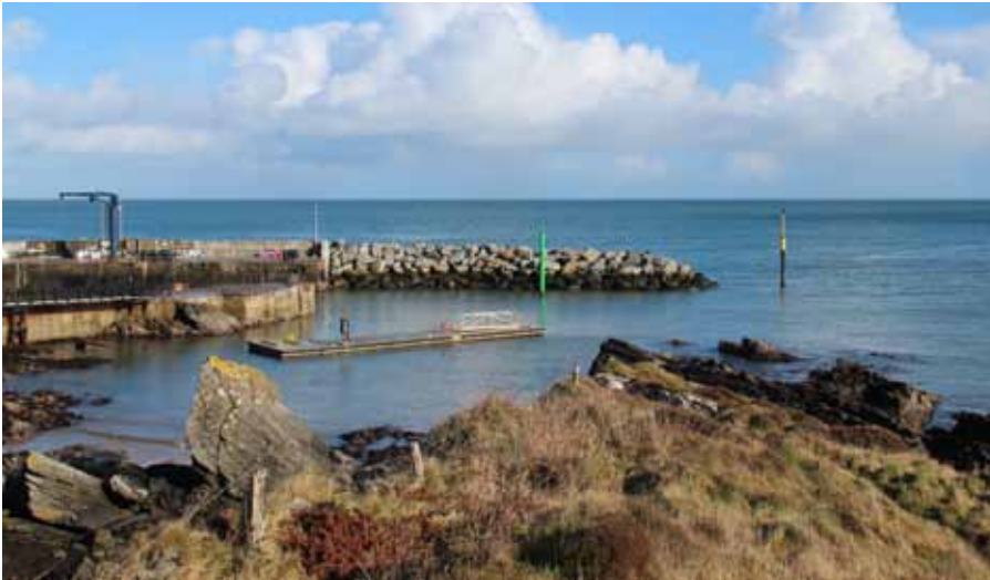
Bunagee in winter condition, February 2016, with only one of the pontoons in position and the gangway swung ashore. The cardinal beacon, R, and the SHM, centre. The PHM is on the other pontoon section, beached for repair.
